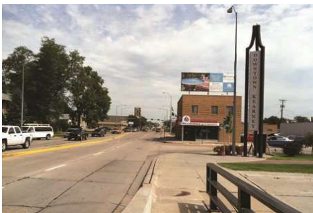
2nd Avenue approaching the 21st Street viaduct landing
