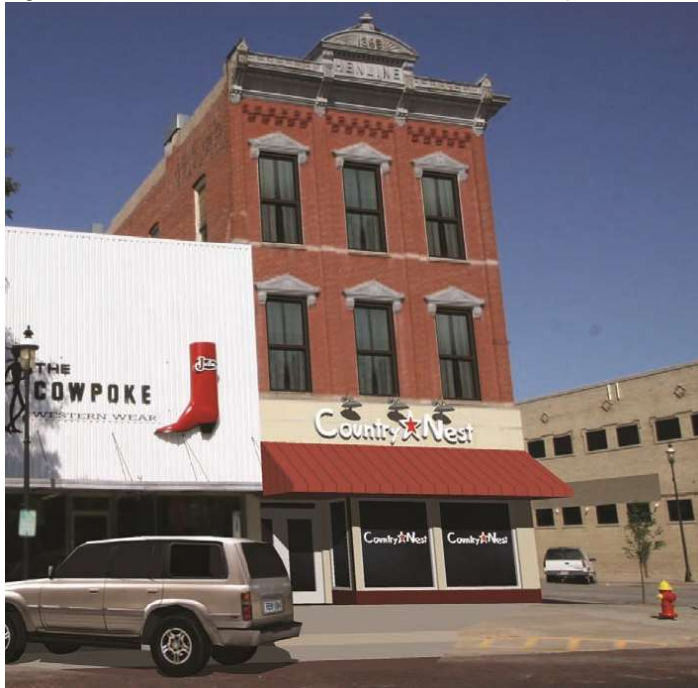
Figure 3.6: Facade Rehabilitation Demonstration - Henline Building
