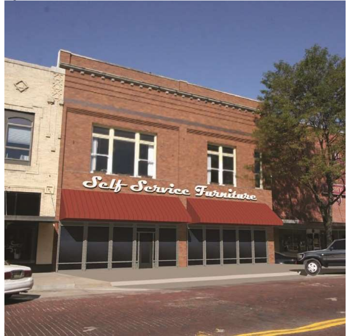
Figure 3.9: Facade Rehabilitation Demonstration - Self Service Furniture
