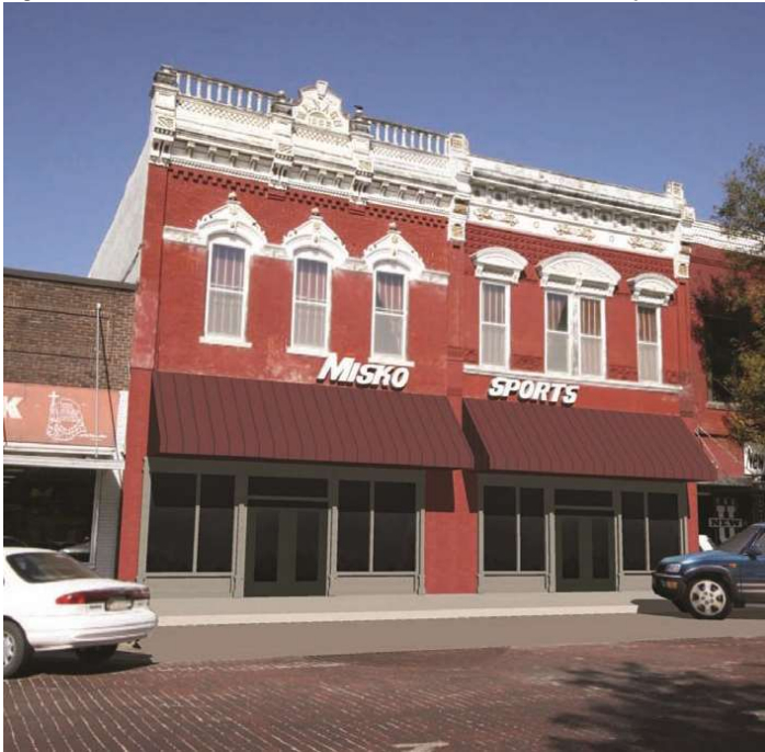
Figure 3.8: Facade Rehabilitation Demonstration - W.L. Nash Building
