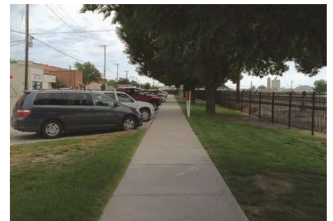
Existing sidewalk near railroad tracks
